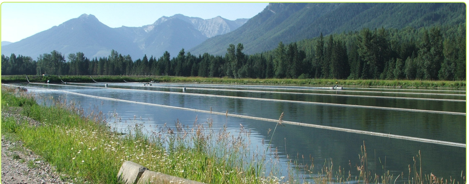
Fernie's sewage treatment lagoons, shown here with newly installed blower lines, currently treat the effluent through 30 to 60 days of aeration. If adopted, the recommended option would see phosphorus reduction and UV disinfection added to the process.
