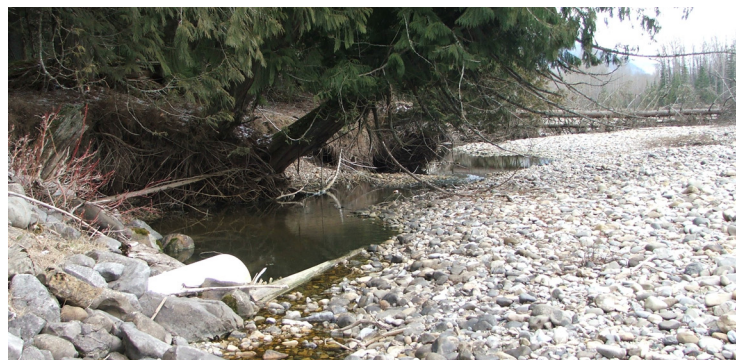
Fernie’s lagoon outfall will need to be moved to the middle of the river to allow proper mixing.
